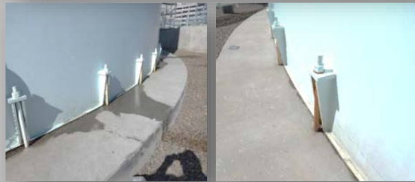
Water at Chime Area.
