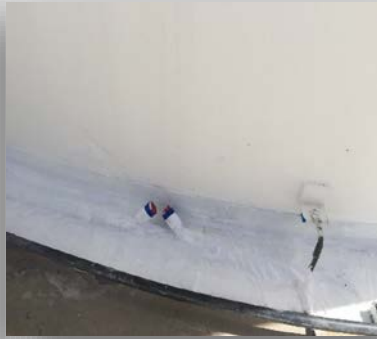
2. Finished installation of Zerust IDS
