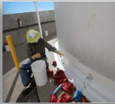
3. Inhibitor slurry injection
