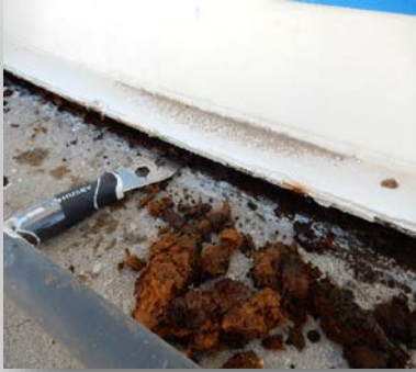
1. Preparation of tank chime & concrete surfaces
