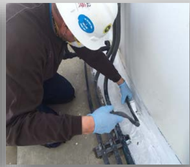
4. Inhibitor sleeves installation
