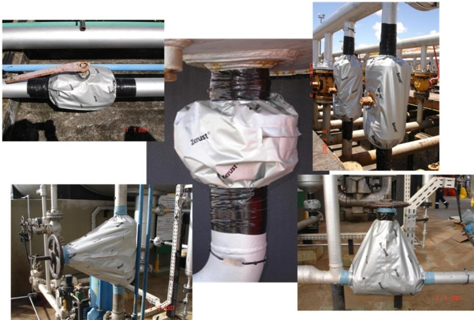
**FIGURE 6 – Various Configurations of FPS Cover Installations**
