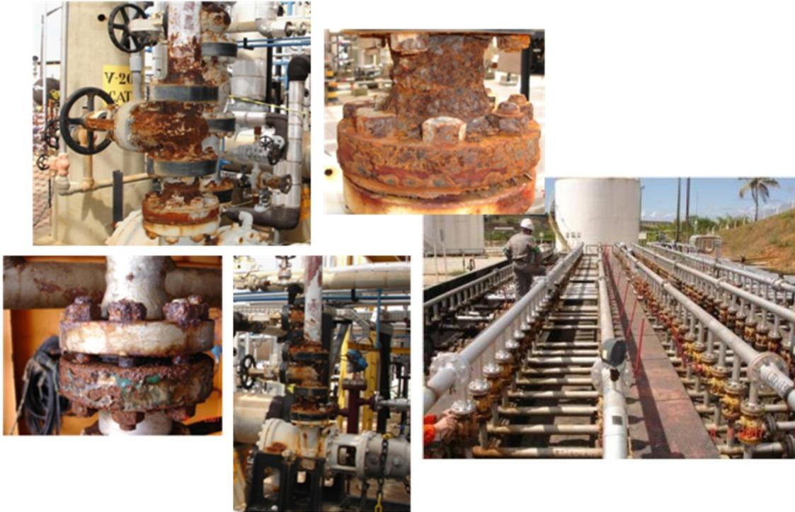
**FIGURE 1 – Examples of Flange corrosion**
