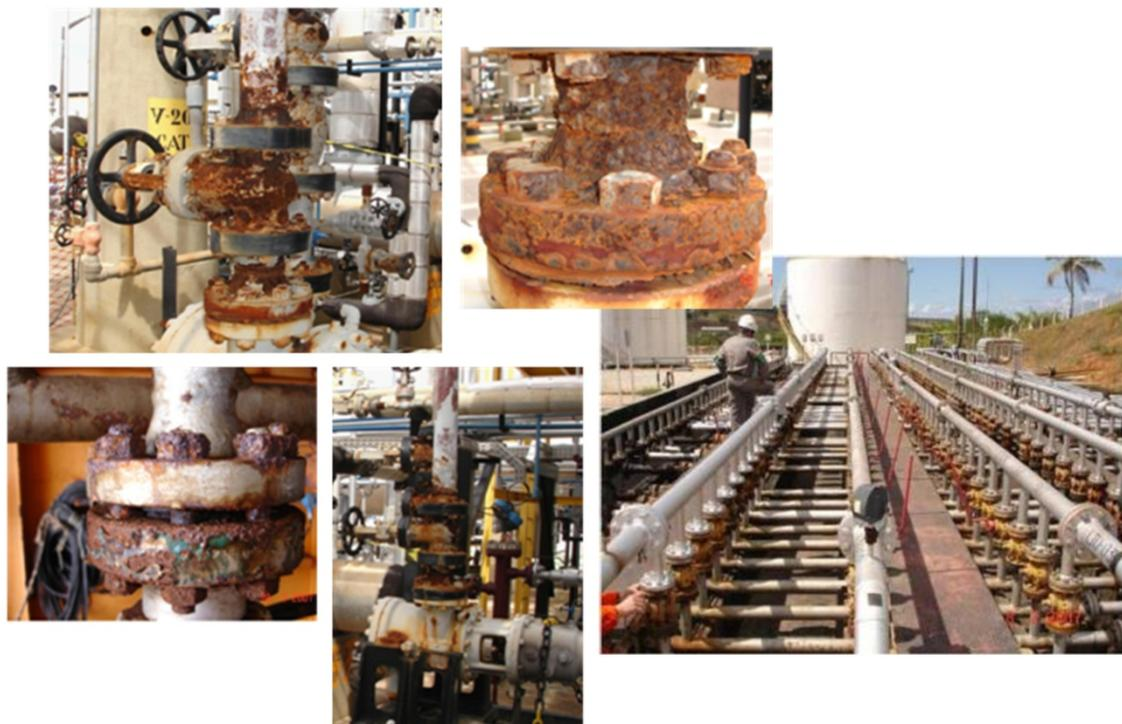
**FIGURE 1 – Examples of Flange corrosion**
