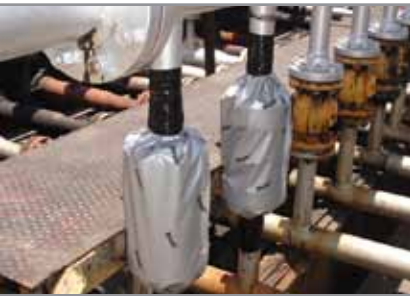
Zerust® Flange Savers™ protect the pipe flanges on the left in a side-by-side field trial.
